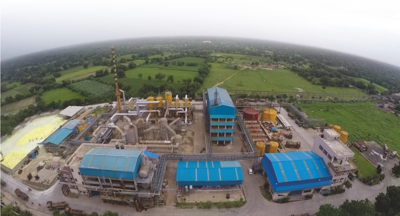
SULPHUR & BULK CHEMICAL DIVISION, VADODARA
